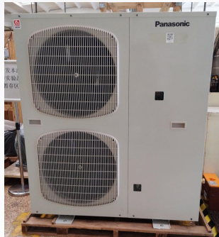
Condensing Unit Outdoor Micro-Channel Series, 3, 4.5, 6 HP Temp. Range -40~+5°C
